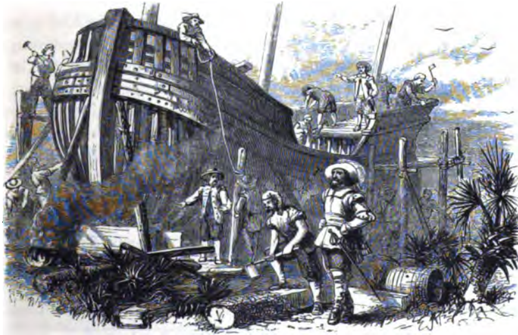
Building the Pinnace.
